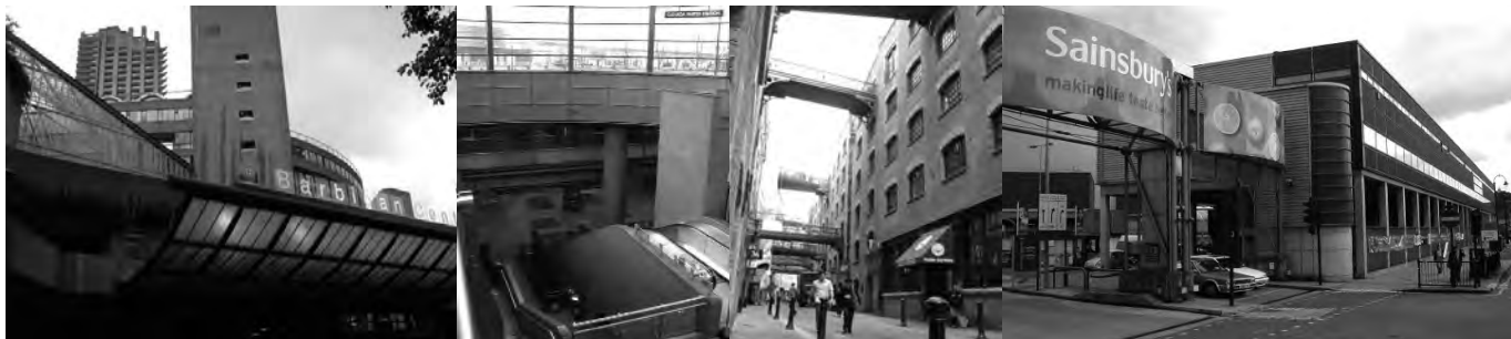
BARBICAN CENTRE_BUTLERS WHARF_BROAD WALL-COIN STREET HOUSING (Haworth Tompkins Architects 2001)_J SAINSBURY'S SUPERMARKET (Nicholas Grimshaw)
