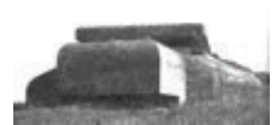
Bunker-two types of facades the upper slab
